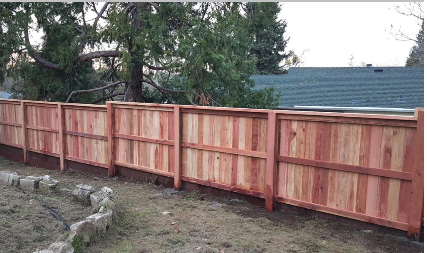
FENCE WITH METAL POSTS WITH FASCIA ADDED
