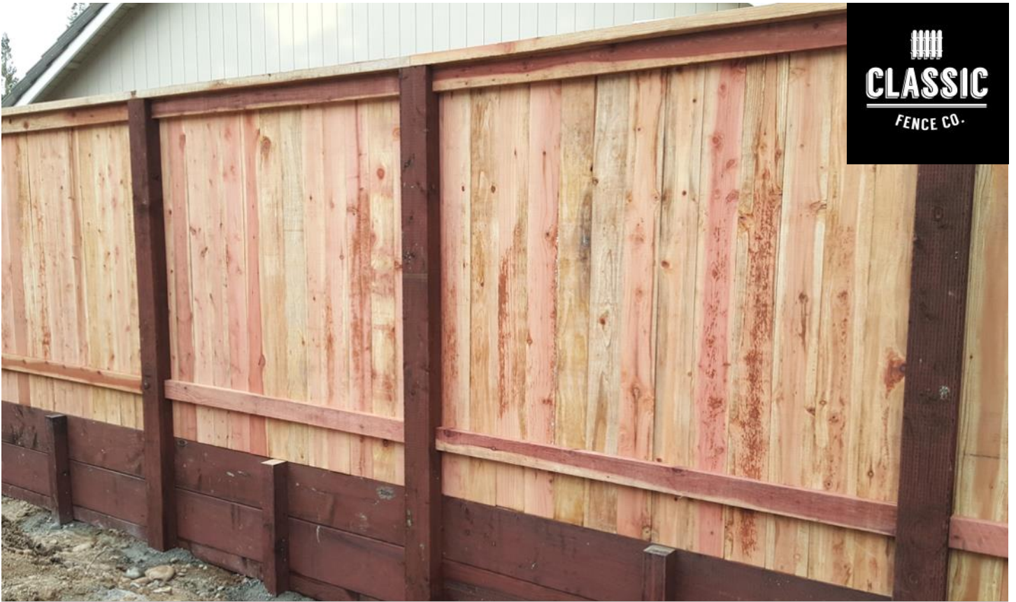
SOLID BOARD WITH 2X6 CAP ON RETAINING WALL - BACK SIDE
