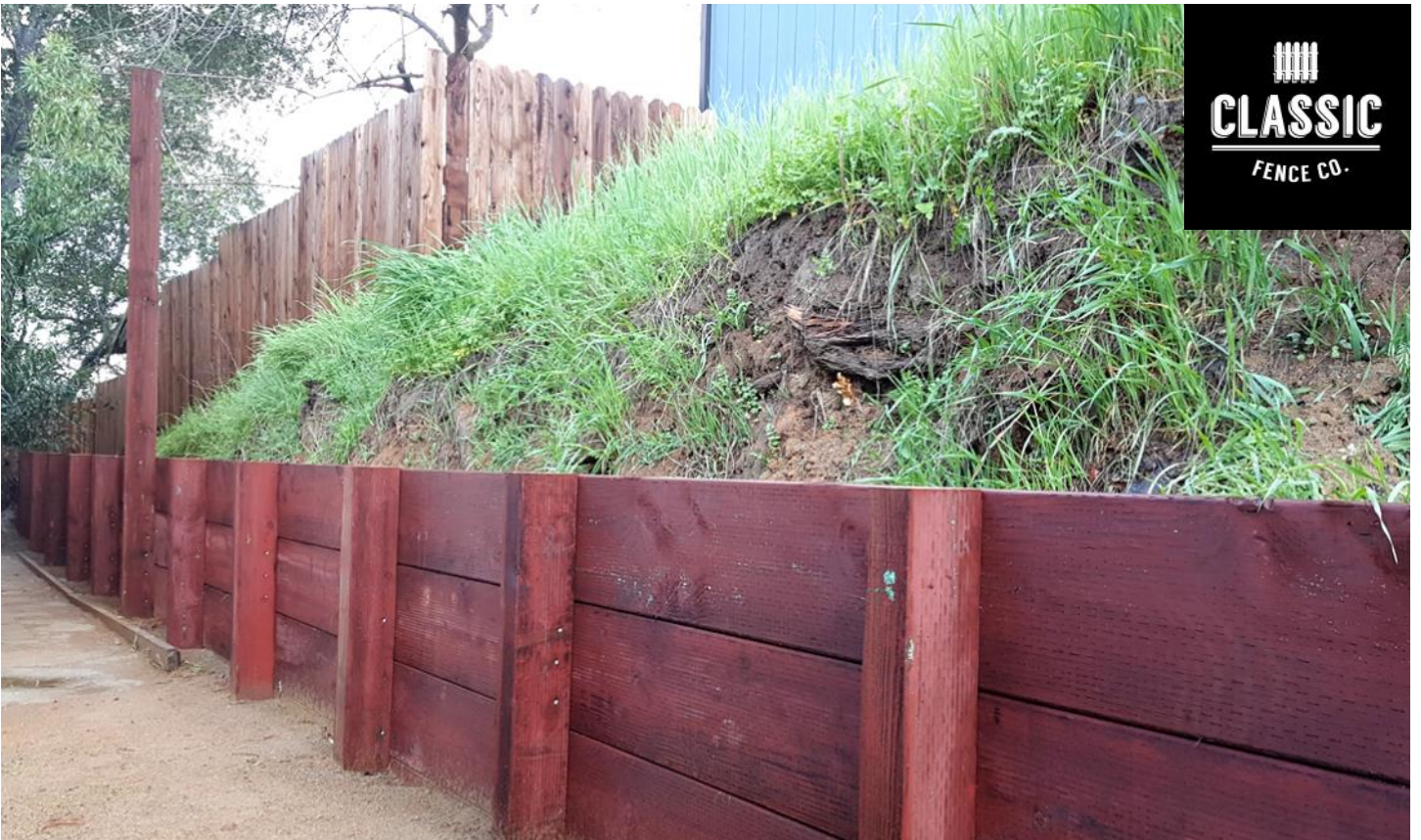
3 FT PRESSURE TREATED DOUGLAS FIR RETAINING WALL
