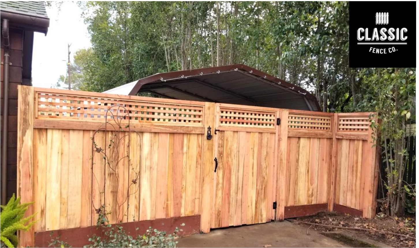
BOARD ON BOARD NAIL ON W/ KICK AND SQUARE PICTURE FRAMED LATTICE
