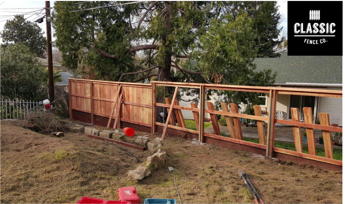
DURING CONSTRUCTION - FENCE WITH METAL POST BEFORE FASCIA ADDED
