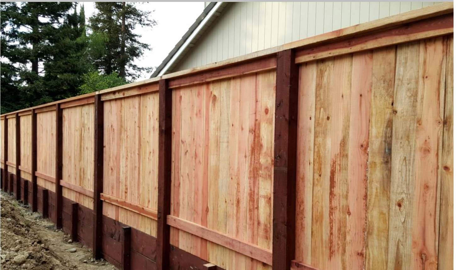
PRESSURE TREATED DOUGLAS FIR RETAINING WALL UNDER FENCE
