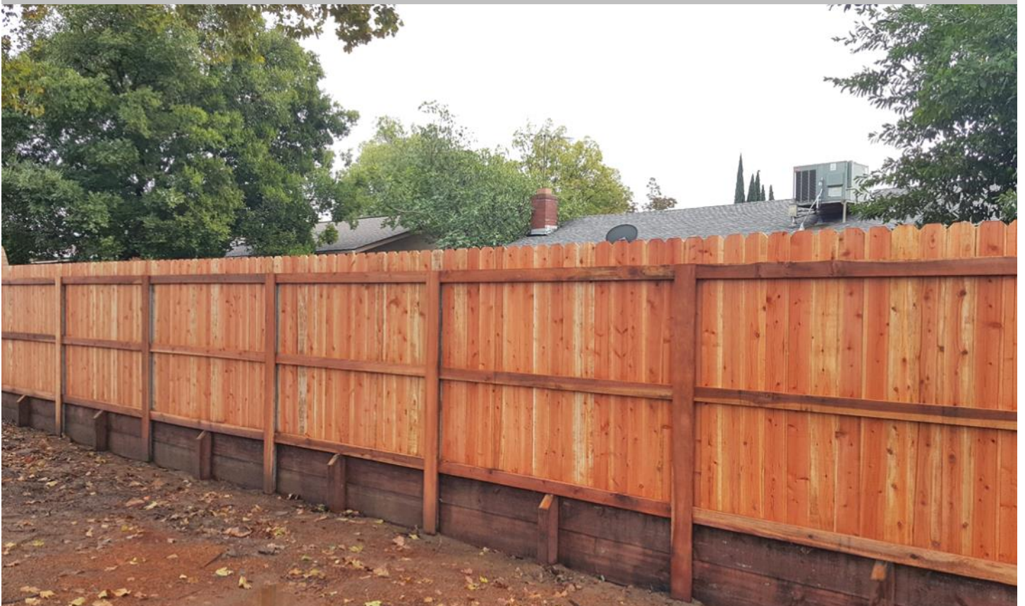
DOGEAR (3) RAIL WITH POSTMASTERS ON RETAINING WALL - BACK SIDE
